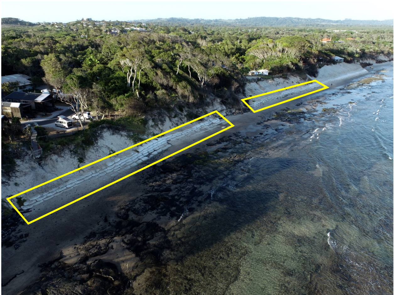
Photo 3 – Existing Reflections Sandbags within the Project Area
